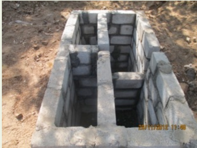
Pits under construction
