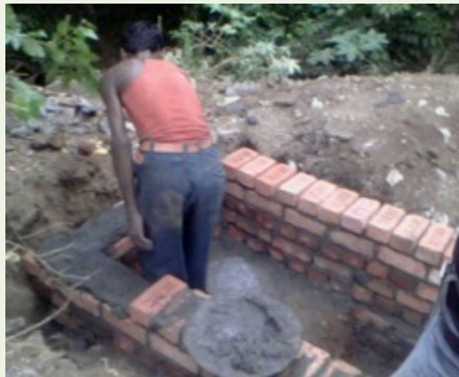
Pits under construction
